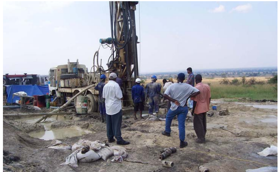
2. Mud drilling at Katwe
