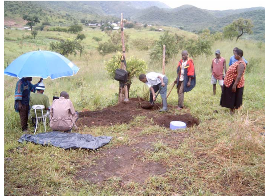
2. Laying an underground sensor
